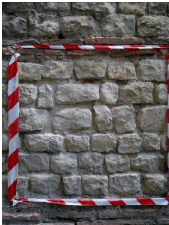
Figure 34 - 1m 2 “time test” area after raking out and re-pointing, east elevation
