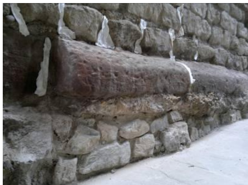
Figure 32 - a) Roman sandstone foundation above modern ground level, east elevation; b) Roman sandstone foundation with lime mortar/ragstone infill to modern ground level, east elevation
