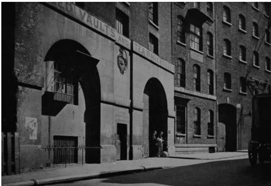
Figure 3 - 'Bonded warehouses in Cooper's Row', image from The City of London: A Record of Destruction and Survival , Corporation of London, 1951, p34
