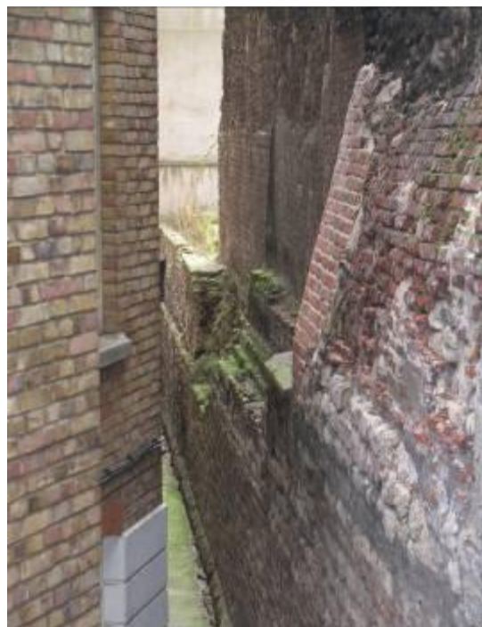
Figure 17 - Looking south along zones M3, M5, east elevation
