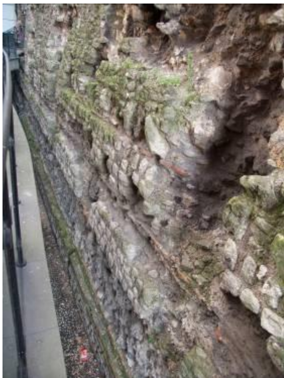
Figure 6 - Looking north along zones R3 - R1, west elevation
