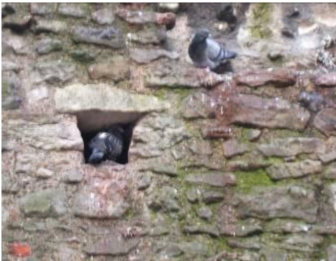
Figure 20 - Pigeons nesting in putlock holes, west elevation
