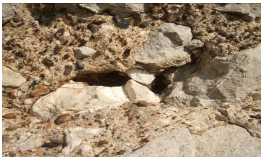
Figure 12 - Detail of cracks between stones and MoW pointing, west elevation
