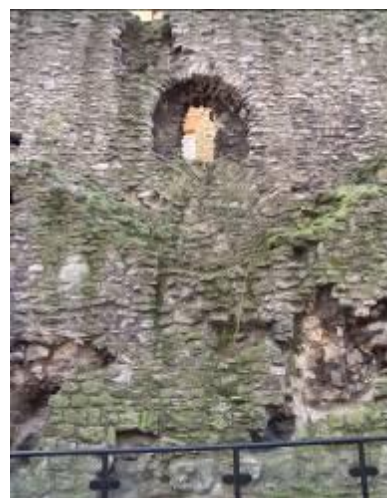
Figure 9 - Zone M3, west elevation
