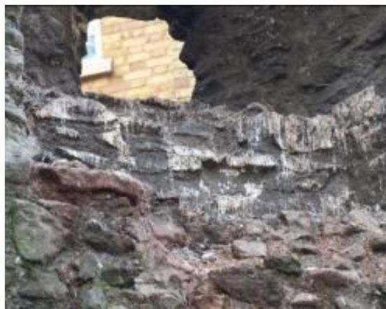
Figure 11 - Detail of M4 opening covered in guano, west elevation
