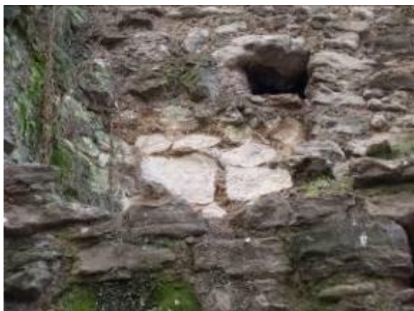
Figure 10 - Detail of M2 showing active chalk decay, plant/bio-infestation and putlock hole, west elevation
