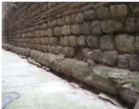
Figure 15 - Looking south along R3 - R5, Roman sandstone foundation, east elevation
