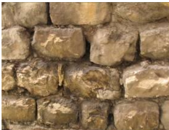
Figure 14 - Detail of pointing losses and voids, east elevation
