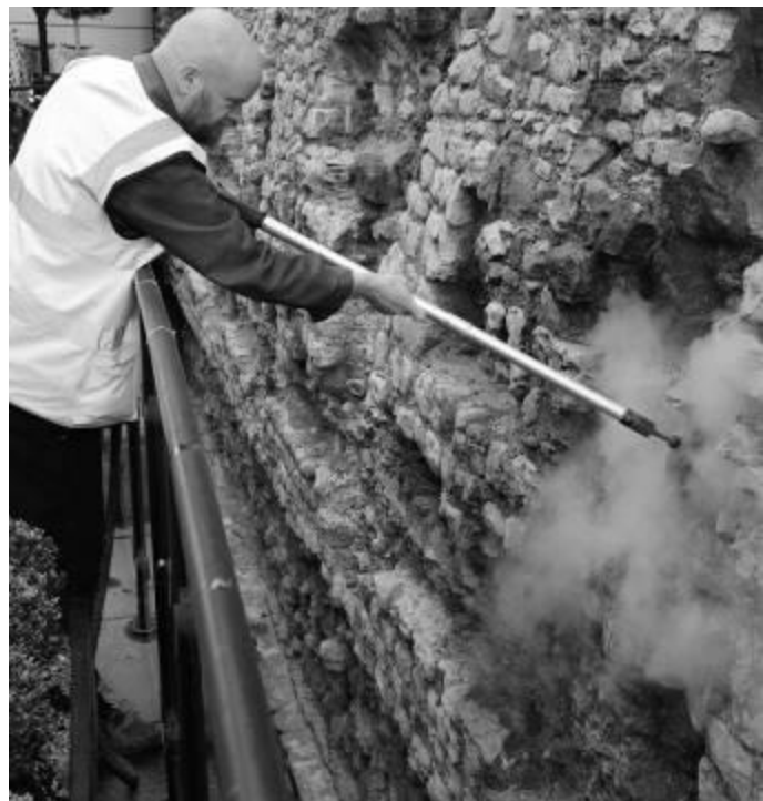
Figure 19 - The author using conservation-grade steam cleaning equipment on the west elevation
