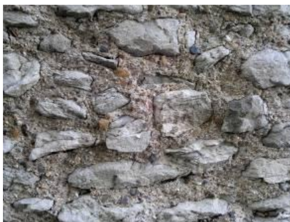
Figure 30 - Minor: losses to ragstone caused by mitigated water egress due to hard cement pointing, west elevation
