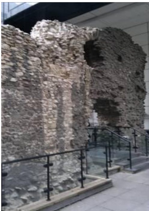
Figure 16 - Looking north along zones M1 - M2, east elevation
