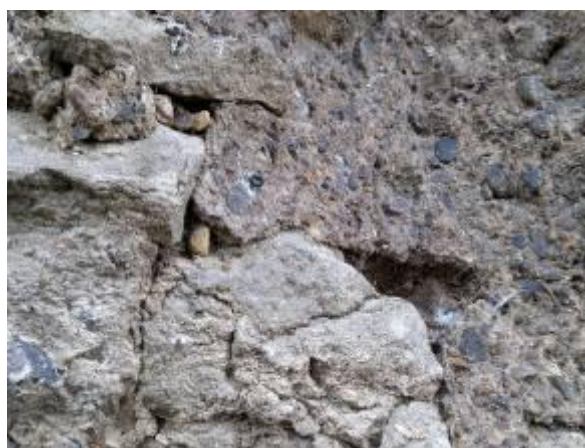
Figure 31 - Significant: losses/voids to/around ragstone due to hard cement pointing inhibiting water egress, west elevation
