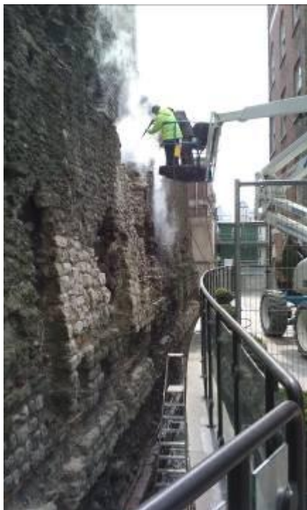
Figure 18 - The author using conservation-grade Thermatech® equipment on the west elevation
