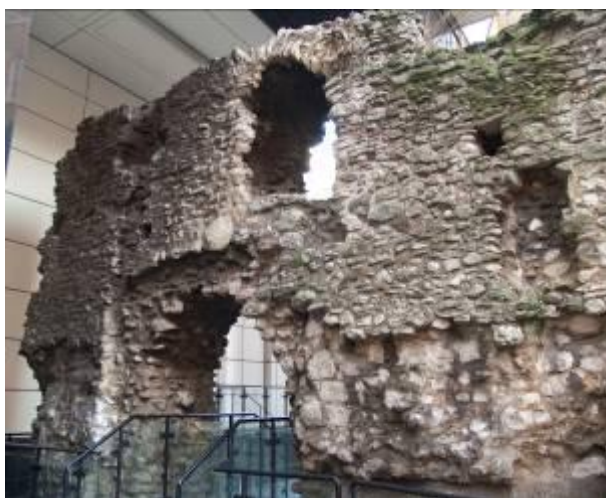
Figure 8 - Looking north along zones M2 - M1, west elevation
