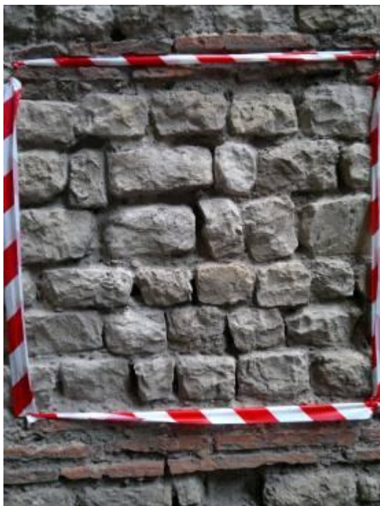
Figure 33 - 1m 2 “time test” area before raking out and re-pointing, east elevation
