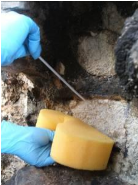
Figure 22 - Applying Calosil E25 by pipette
