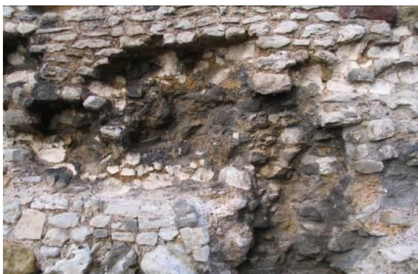
Figure 13 - Detail of chalk decay, sulphation and MoW cement pointing, zone M3, west elevation
