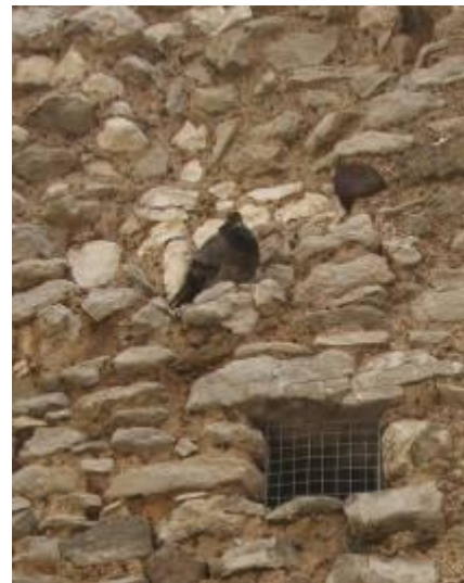
Figure 21 - Pigeons denied access to putlock holes by galvanised wire cages, west elevation
